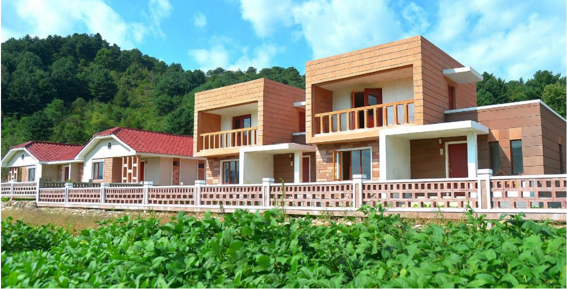
Some of dwelling houses newly-built in the rural areas throughout the country
